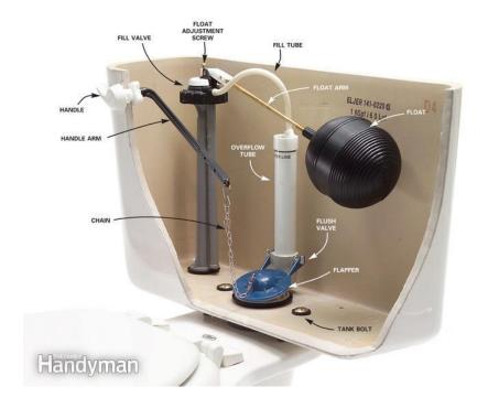
The flush function is the one that can impinge on your daily routine when it malfunctions. The flush system consists of the trip lever and the flush valve. When you push the trip lever, it lifts the flush valve (a.k.a. the flapper) which floats while the tank empties into the bowl. When the tank is empty the flush valve settles onto its seat, then water intake valve opens to refill the tank.
